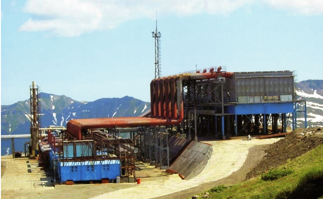
Fig. 4. Verhkne-Mutnovsky (Russia) 12 MW flash-steam plant with ACCs. Photo from Geothermal Power Plants, 2 nd . Ed. , 2008 by R. DiPippo.
